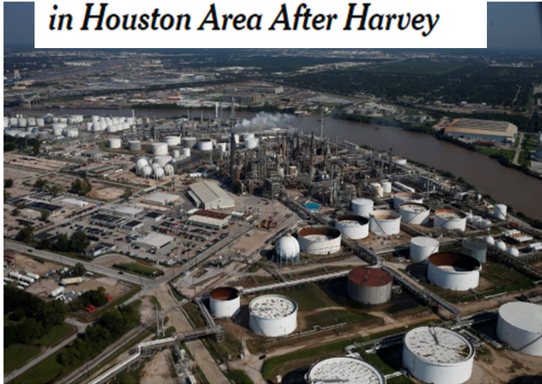
An aerial view of the Valero Houston Refinery is seen in Houston, Texas, U.S. August 31, 2017. REUTERS/Adrees Latif Published Credit: adrees latif/Reuters PHOTO: ADREES LATIF/REUTERS
